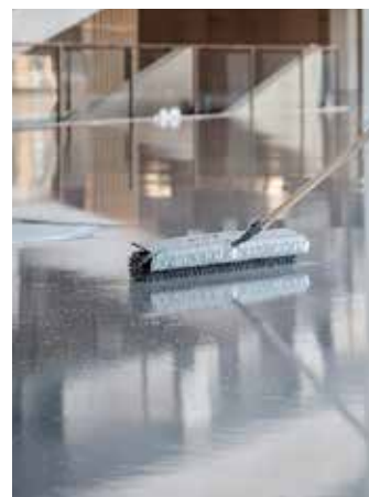
6. Apply UZIN NC 195 with a thickness of approximately 8 mm
