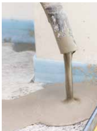
5. Application of thin screed UZIN NC 195
