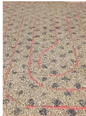
3. Flat deduction of SYMPOR-LB 400 (or Sympor LB 400 S) directly at the top edge of the nubs
