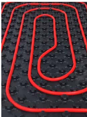
1. Installation of Sympor Unisolo 14-17 on a clean surface. Insertion of floor heating pipes
